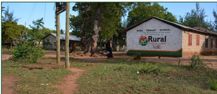
Bowa Rural Electrification Project, Matuga Constituency - Kwale County
