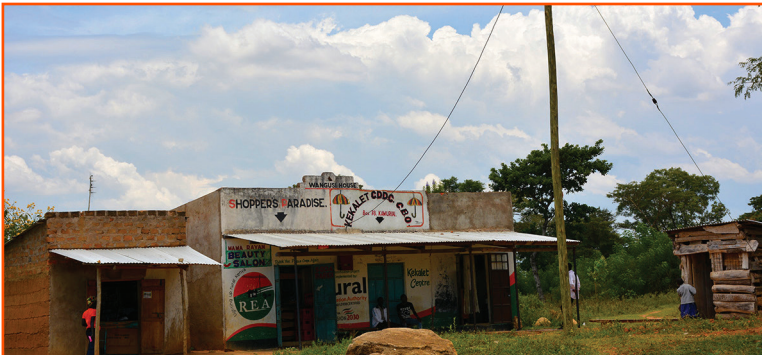
Kekalet Rural Electrification Project, Teso North Constituency - Busia County
